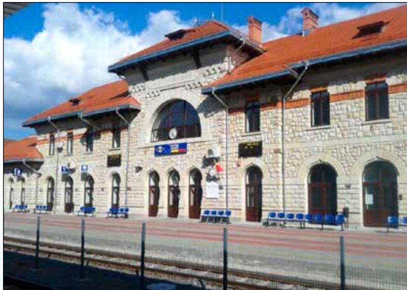
Building of Piatra Neamț railway station (Romania) after modernization
