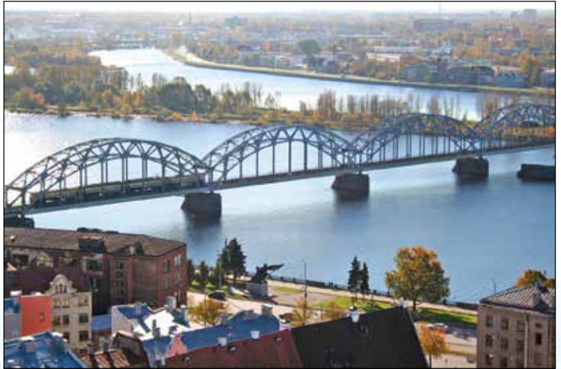
Railway bridge in Riga (LDZ)
