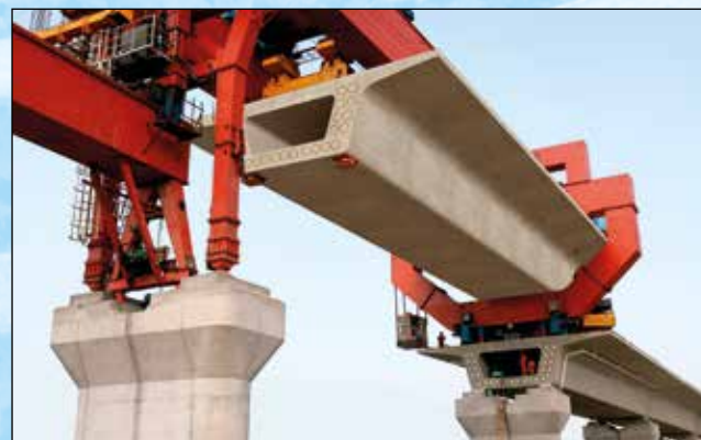
Mounting of a free-support balk of 900 tons in weight and 32 m in length on a high-speed line of the Chinese Railways
