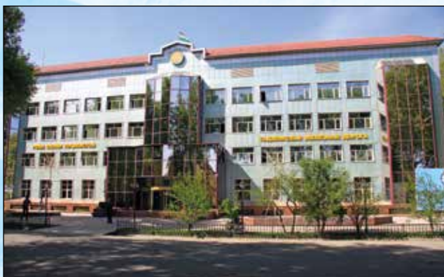
Administrative Building of SUE "ROT" (Railway of Tajikistan) in Dushanbe
