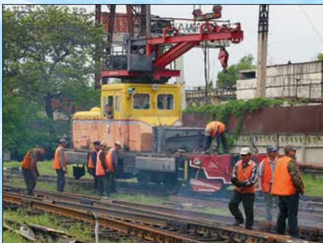
Track maintenance works on the Kyrgyzstan's Railway
