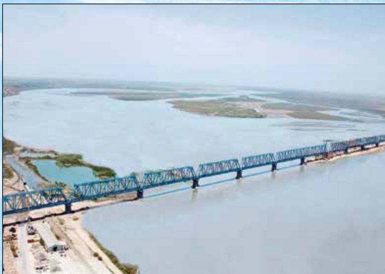
Railway bridge over the Amu-Darya river on the new line Turkmenabat – Atamurat – Kerkechi (Turkmenistan)
