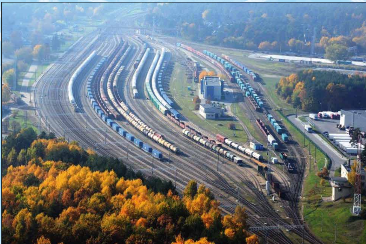
Vaidotai Station (Lithuanian Railways) is the first fully automated sorting railway station in Eastern Europe
