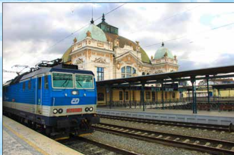
Railway station in Pilsen (Czech Railways) after modernisation
