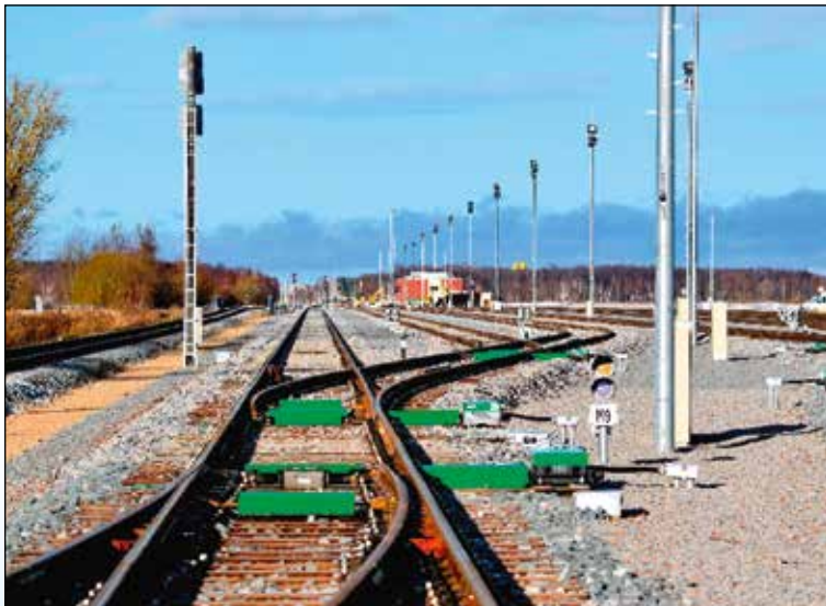
Bolderāja-2 railway station (Latvian Railway) after completion of the modernisation project
