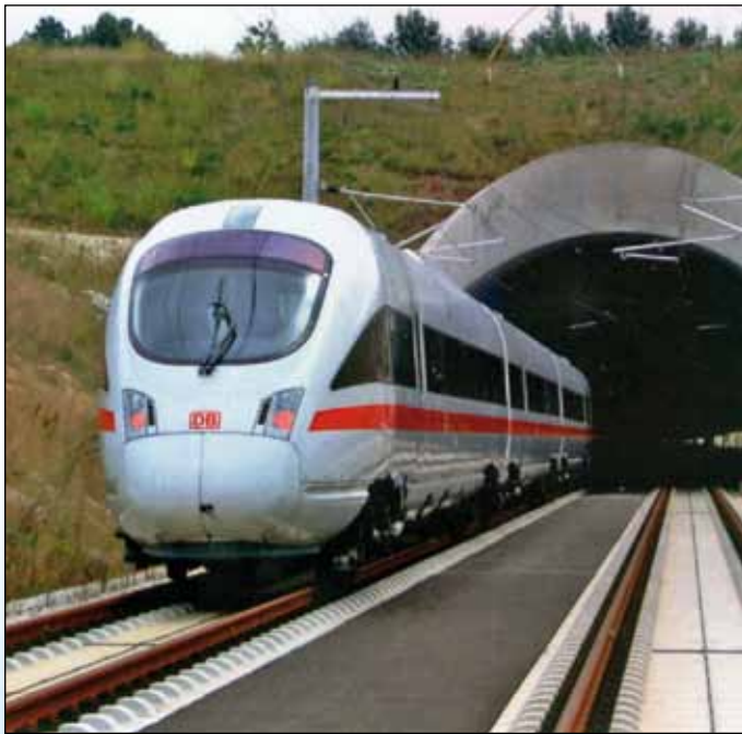
Nürnberg - Ingolstadt section of an ICE high-speed railway line of DB AG (OSJD observer), built by Max Bögl (OSJD affiliated enterprise, Germany)
