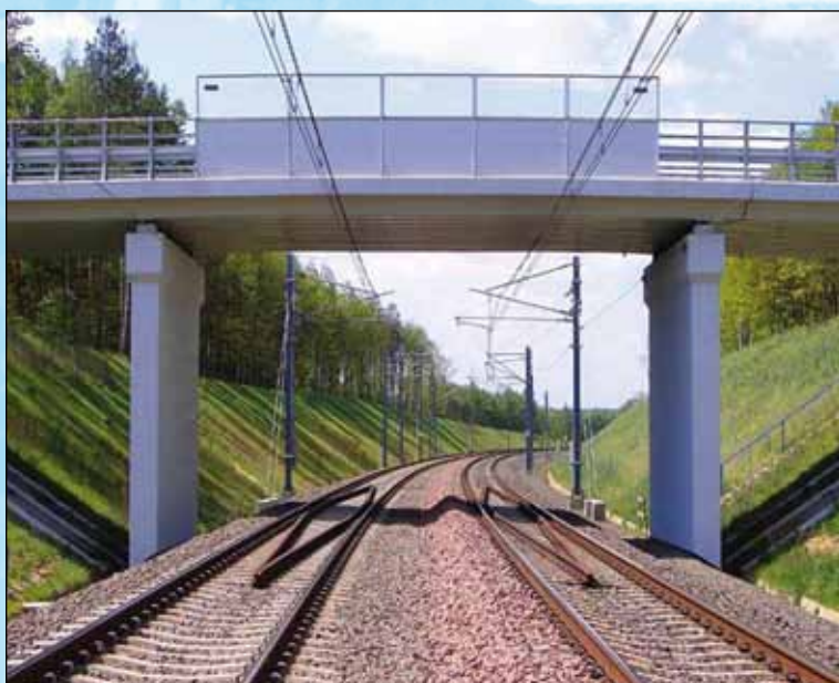
Chojnow – Okmiany railway section for fast traffic (Polish State Railways – PKP)
