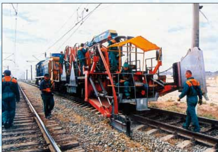
Repair works at Azerbaijani Railways
