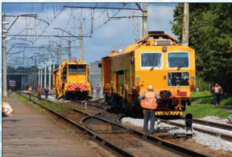
Engineering works at Latvian Railway (LDZ)
