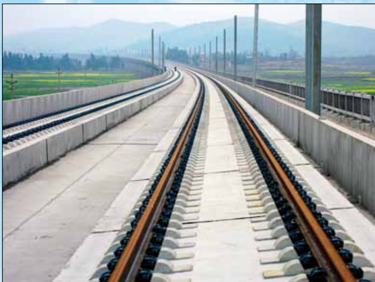
One of the KZD high-speed railway lines being built in China
