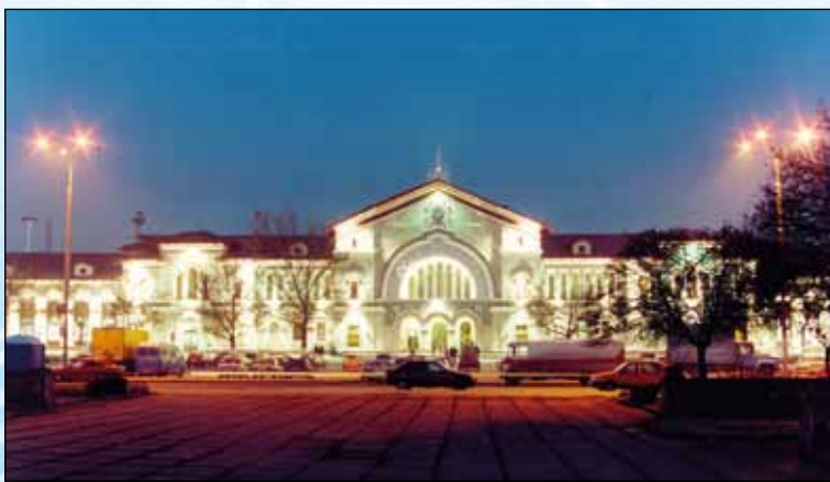
Railway station in Chişinău after reconstruction (Railway of Moldova)
